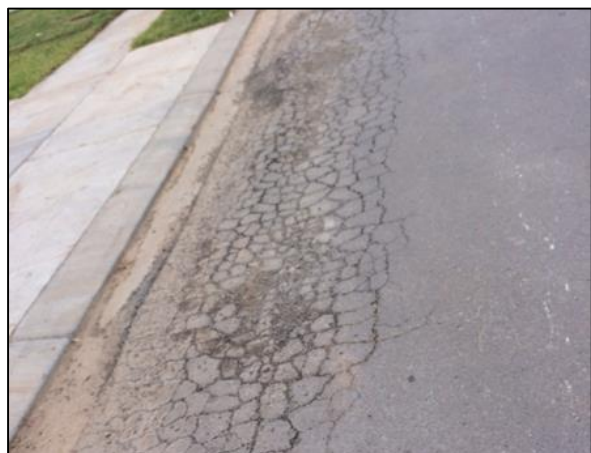
Figure 8: Baker Meadow Alligator Cracking
