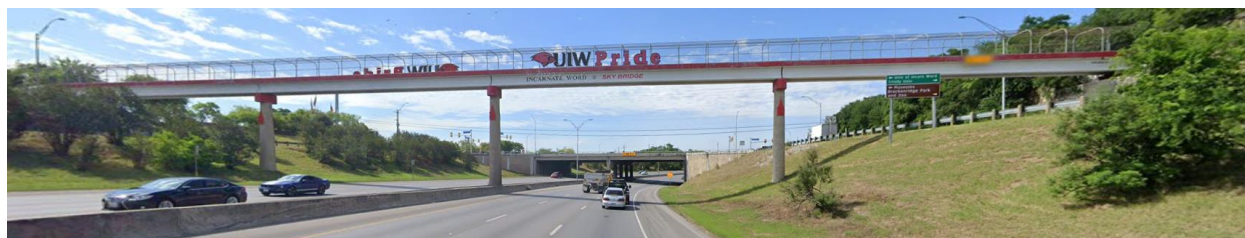
Figure 4: Pedestrian Bridge over US 281 in San Antonio (Source: Google Street View)
