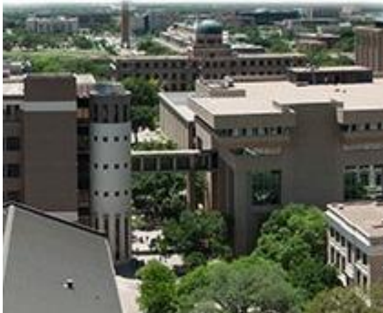
Figure 11: “Skywalk” between Evans Library and the Annex
