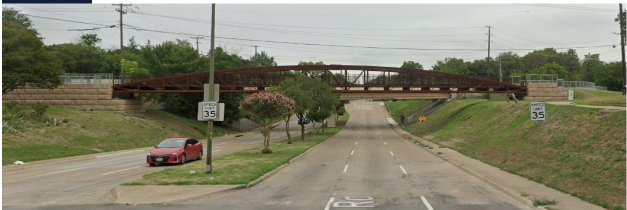
Figure 9: Abrams Rd Depressed Below Ridgewood Trail in Dallas (Source: Google Street View)
