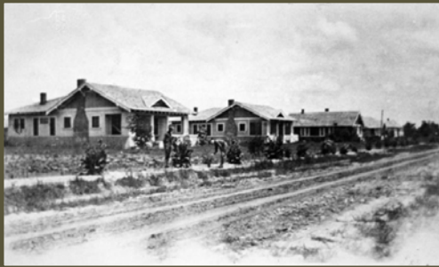
Figure 1.3 Campus Homes Source: Photo-Project Hold.
