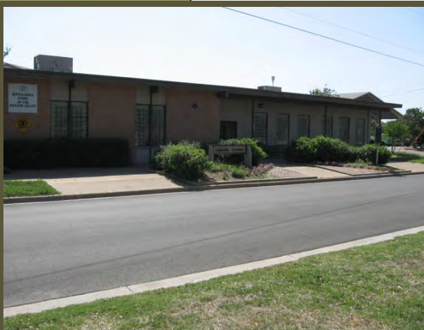
Figure 4.1 Lincoln Center. Source: Neighborhood Resource Team
