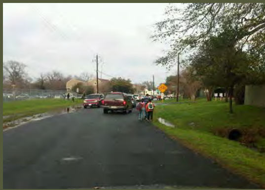
Figure 4.4 Open ditch drainage limits pedestrian accessibility.
