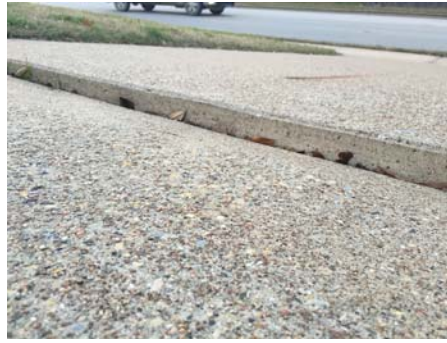
AR Violation 12 - The sidewalk in front of the pool facility that connects to the sidewalk along Rock Prairie Road has significant level changes.
