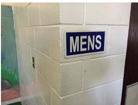
Hallway Violation 3 - The room signs within the park facilities are not accessible. Many do not include tactile characters or Braille.
