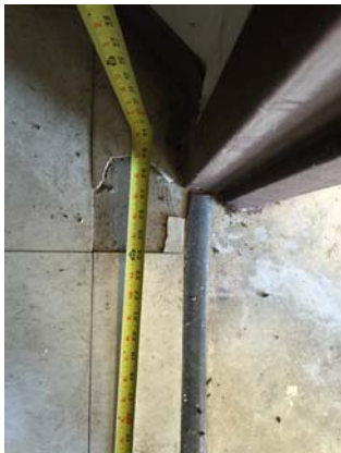
Hallway Violation 1 - The doors into the concessions areas provide only 27" clear width where 32" minimum is required.
