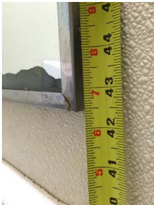
RR Violation 8 - The mirrors in the men's and women's restrooms serving the tennis courts are mounted above 40" to the bottom of the reflecting surface.
