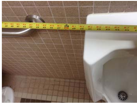
RR Violation 16 - Men Restroom 254 - The clearance between the water closet sidewall and the urinal is 50-1/2". The water closet must have a 60" minimum clearance from the sidewall. At the time of construction 2002/2003 the only fixture permitted to be within the 60" minimum clearance was a lavatory.
