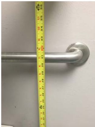
RR Violation 4 - The grab bars within the Southwood Community Center restrooms are too low at 31-1/2" to the top of the bars.
