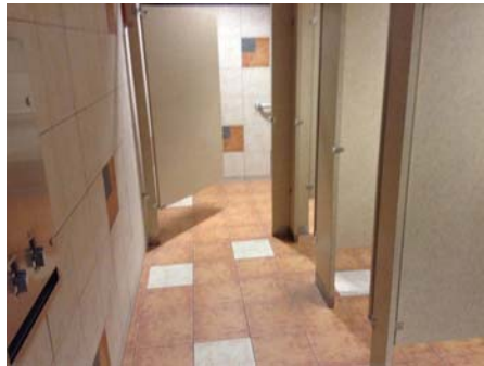
RR Violation 9 - 1st floor Women Restroom (Fire Admin) - The door into the accessible toilet compartment does not self-close.
