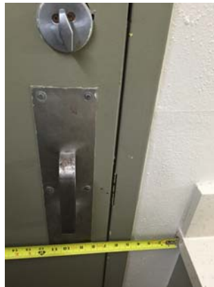
Hallway Violation 2 - The doors within the pavilion do not have the required 18" clearance on the pull side of the doors.
