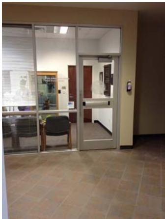
Hallway Violation 1 - The room identification at the the Fire Administration/Fire Prevention office area is etched into the glass adjacent to the the door. Signs designating permanent spaces must be accessible and include raised tactile characters and Braille.
