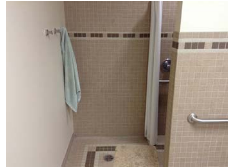
RR Violation 17 - Men Restroom 254 - The wall mounted hooks next to the shower are installed at 60" above the floor. At least one hook must be provided at 48" high.
