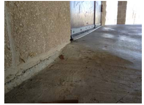
Entrance Violation 1 - The entrance door into the pool house has a 7% slope on the exterior of the door where it is required to be level.
