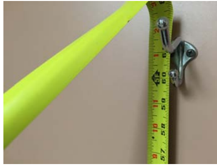
RR Violation 3 - The coat hook in the accessible stall in both the men's and women's restrooms are mounted at 60" above the finished floor.
