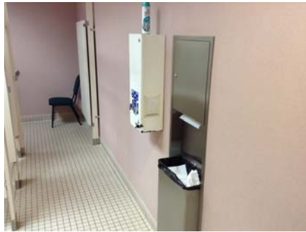
RR Violation 5 - Employee Women Restroom -The surface mounted feminine product dispenser is a protruding object as it extends 8" from the wall into the circulation path to the accessible toilet compartment.
