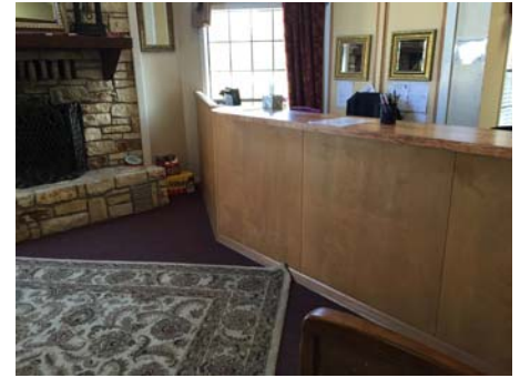
Misc Violation 2 - The main counter in the lobby has a height of 45" high with no lowered section.
