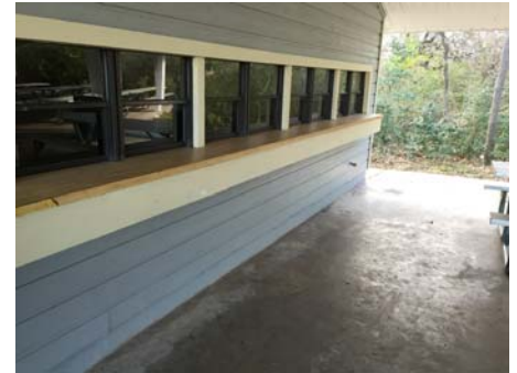
Park Violation 3 - The concession stand attached to the Rec building has counters that are 42" high with no lowered counter.
