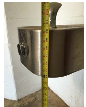
Misc Violation 2 - Only one drinking fountain is provided at each little league field complex. The units that are provided only have 24" knee clearance where 27" minimum is required. No drinking fountains for standing persons are provided.
