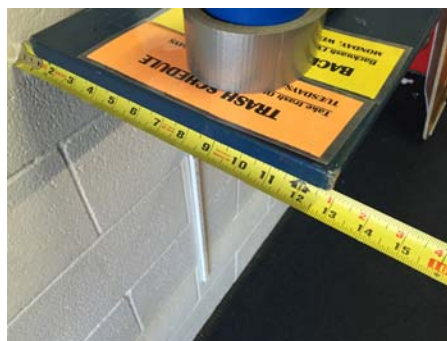
Hallway Violation 4 - The wall mounted shelving within the interior of the pool house is a protruding object.
