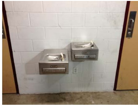
Misc Violation 1 - The high drinking fountain located between the restrooms is a protruding object.
