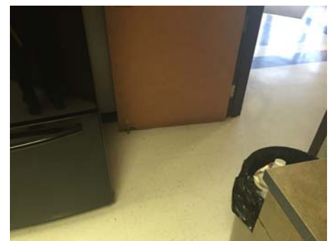
Hallway Violation 5 - The width of the route into the Southwood Community Center staff break room is only 29" between the refrigerator and the countertop.
