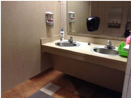
RR Violation 8 - 1st floor Women Restroom (Fire Admin) - The soap dispensers located above the lavatory counter are 49" above the floor. Accessible reach range over an obstruction is 44" maximum.
