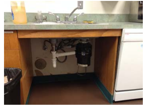
BR Violation 1,2 - Employee Lunchroom - The garbage disposal obstructs the required knee clearance under the sink. At the time of construction of this facility, a knee/toe clearance for a forward approach was required. The exposed water lines and drain pipe are not protected against contact.
