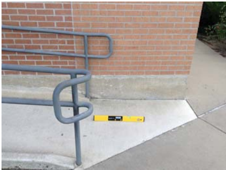
AR Violation 2 - The exterior ramp that provides access up to the north side main entrance has a running slope of 4% and a cross slope of 2.7% within the landing area at the bottom of the ramp. Ramp landings must have a cross slope of 1:48 maximum in all directions.
