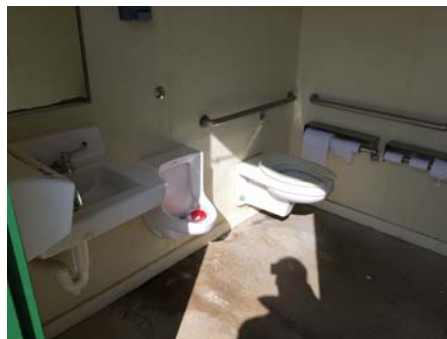
RR Violation 9 - The urinal is not permitted to be located within 60" of the water closet sidewall.
