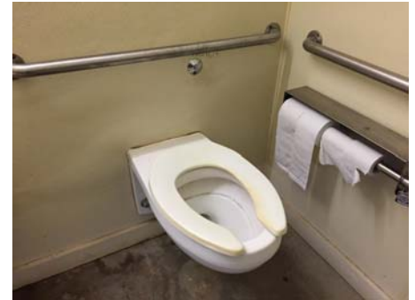
RR Violation 7 - The men's room serving the tennis courts has the flush control on the wrong side.
