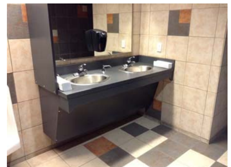
RR Violation 2 - 1st floor Lobby Men Restroom - The soap dispenser located above the lavatory counter is 50" above the floor. Accessible reach range over an obstruction is 44" maximum.
