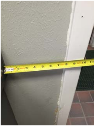
Break Room Violation 2 - The door maneuvering clearance for the break room door is only 10" on the pull side of the door. 18" is required.
