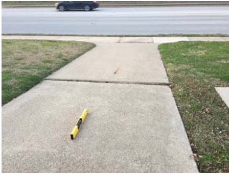
AR Violation 12 - The sidewalk in front of the pool facility that connects to the sidewalk along Rock Prairie Road has a running slope of 12%.
