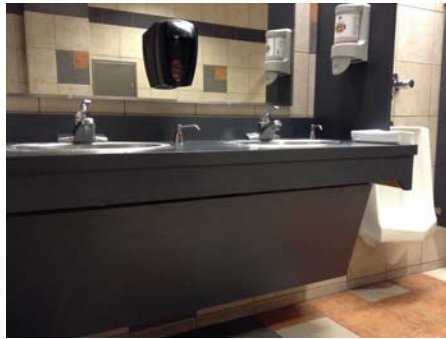
RR Violation 6 - 1st floor Men Restroom (Fire Admin) - The soap dispensers located above the lavatory counter are 49" above the floor. Accessible reach range over an obstruction is 44" maximum.
