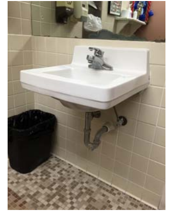
RR Violation 4 - The pipes underneath the lavatories in both the men's and women's restrooms, on both floors, are not wrapped or protected from contact.
