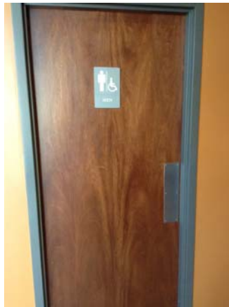
RR Violation 1,5 - 1st floor lobby Men Restroom - The room sign is located on the door where it is required to be installed on the latch side of the door.
