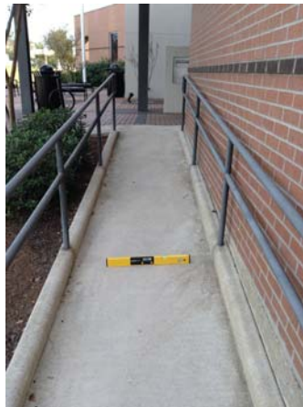
AR Violation 3 - The exterior ramp that provides access up to the north side main entrance has a cross slope of 3.8% within the ramp segment. The ramp must have a cross slope not exceeding 1:48 throughout its length.
