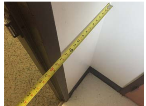
Hallway Violation 2 - Within the Southwood Community Center the doors in the restroom corridor have 16" of clearance on the pull side of the doors.
