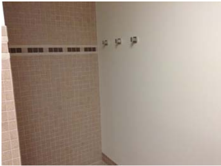
RR Violation 15 - Women Restroom 255 - The wall mounted hooks next to the shower are installed at 60" above the floor. At least one hook must be provided at 48" high.
